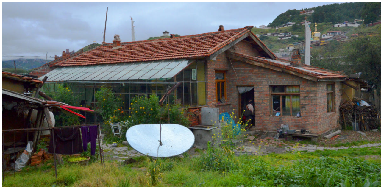
Figure 22: Solar stoves and glassed porches are in common use in the Tibetan areas to make use of the sun light
